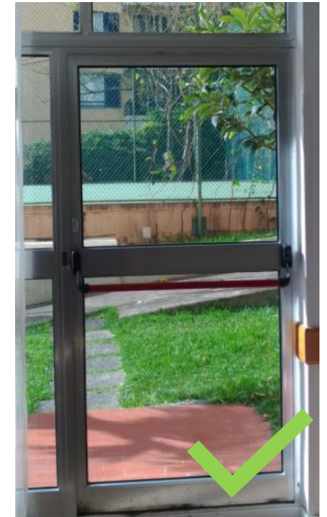
Push Bar Installed
